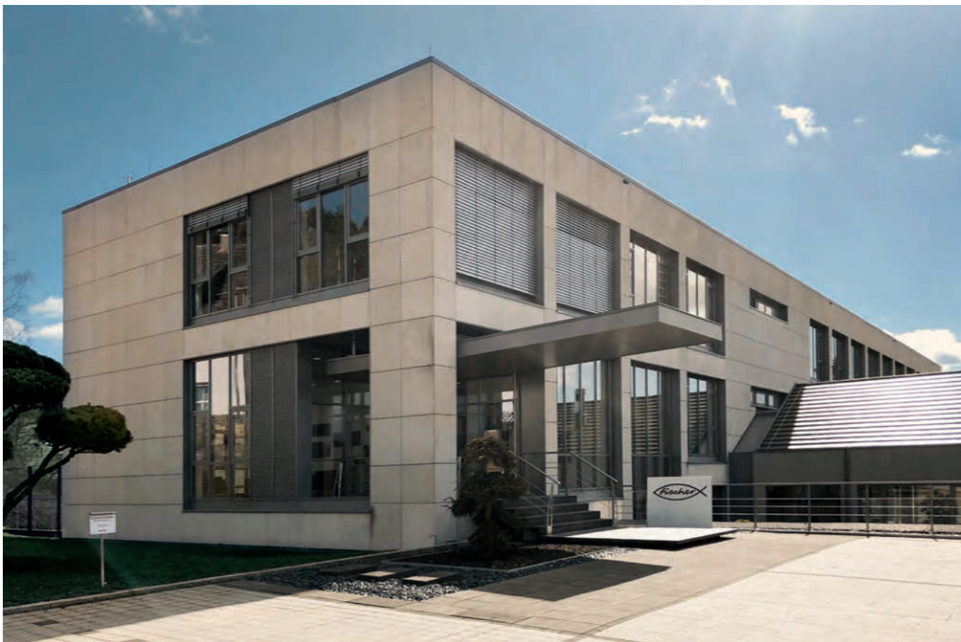
fischer administration building · Waldachtal · Germany
