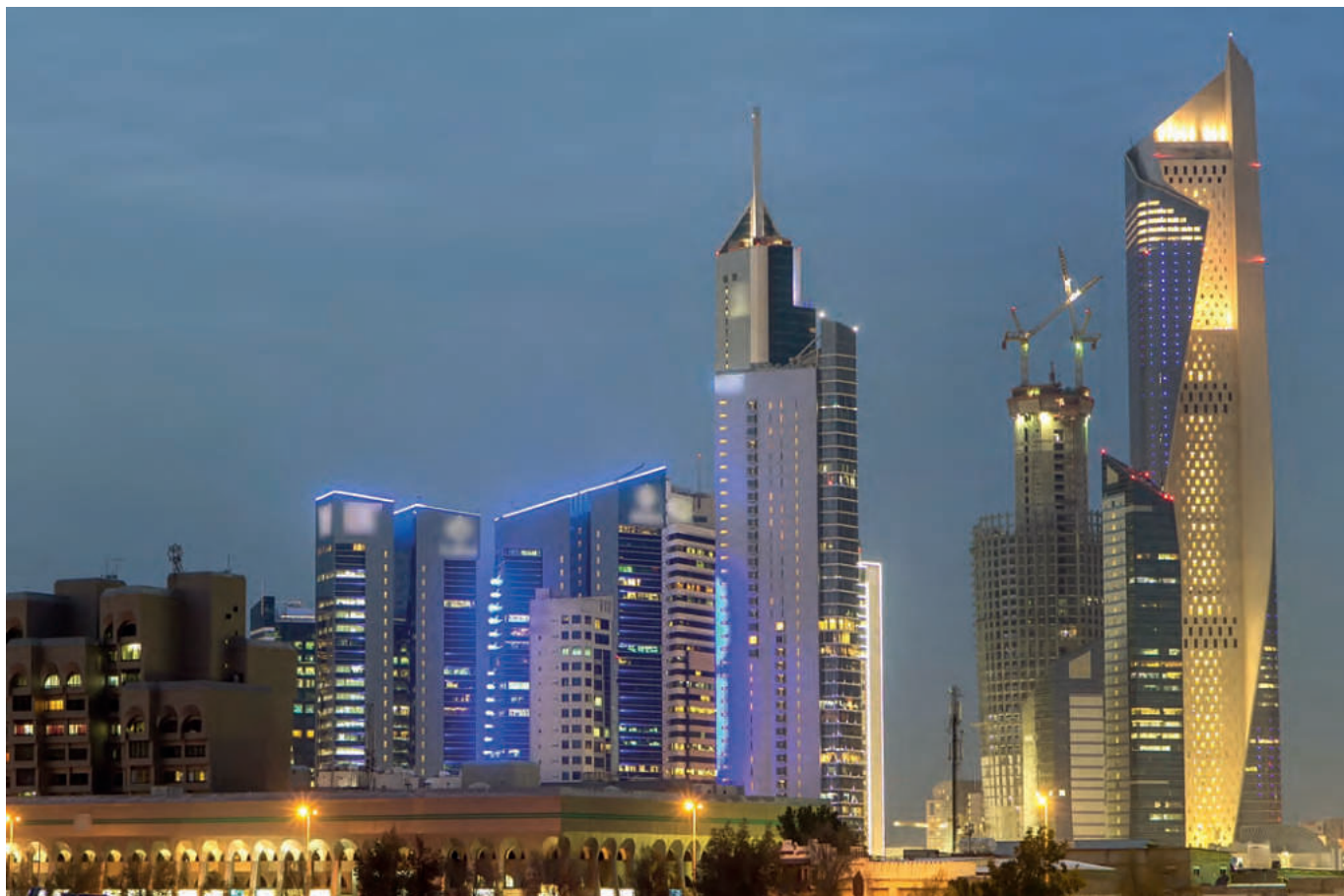
Al Hamra Tower · Kuwait
