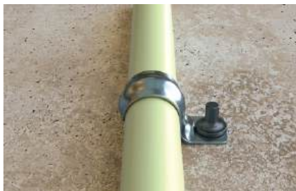
Fixing armoured conduits
