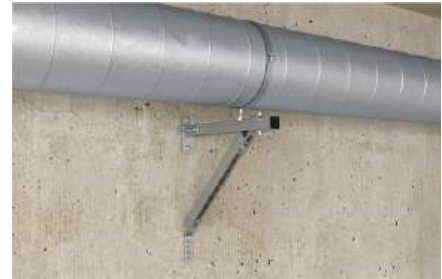
Spiral airduct on cantilever
