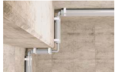
Fixing plastic insulating conduits
