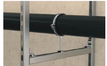
Pipe fixing on frame construction
