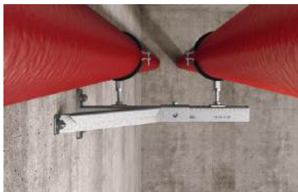
Bracing of cantilever construction
