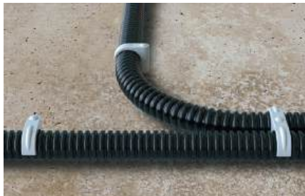
Fixing flexible pipes
