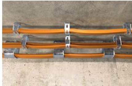
Cable fixing to the ceiling
