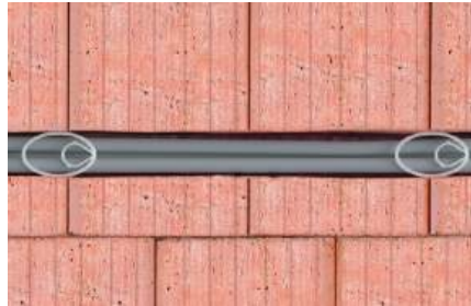
Cable fixing in wall slots > 30 mm
