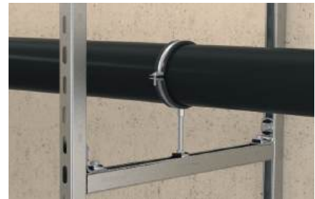
Pipe fixing on frame construction
