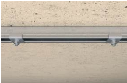
Channel installation at ceiling
