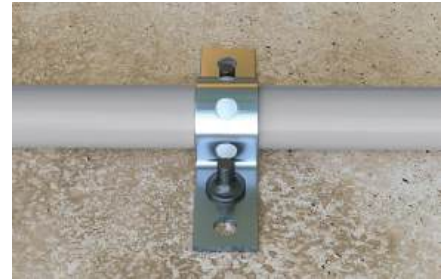
Fixing perforated tapes
