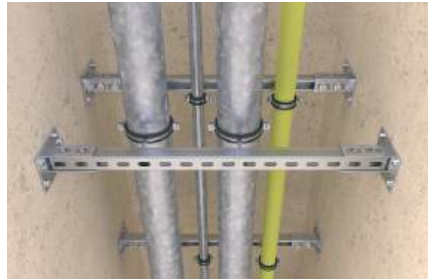
Pipe installation in escape route
