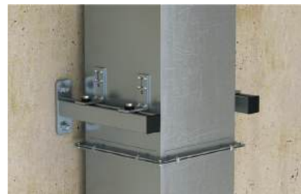
Air duct vertical installation utilising LKHS
