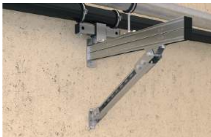
Massive bracing of cantilever arm
