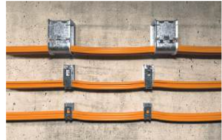
Cable fixing to the wall
