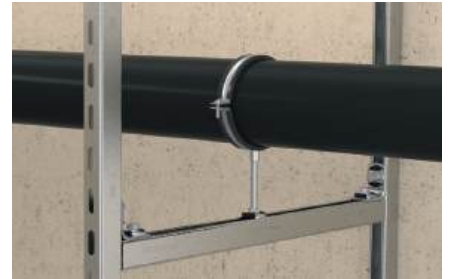
Pipe fixing on frame construction
