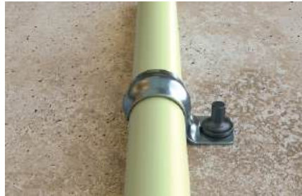
Fixing armoured conduits
