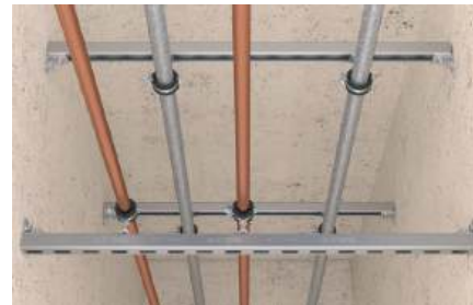
Pipe fixing in a corridor
