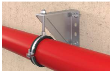
Heavy drainage pipe under angle bracket
