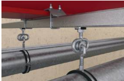
Channel fixing to steel beam
