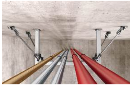
Bracing of frame construction with threaded rods
