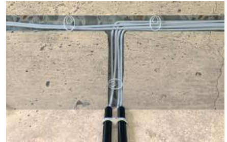
Cable fixing in wall slots < 55 mm
