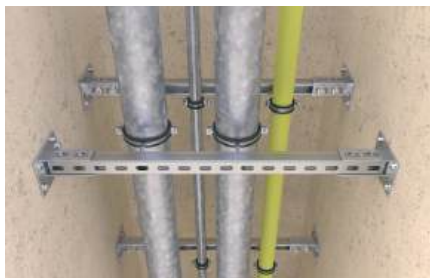
Pipe installation in escape route
