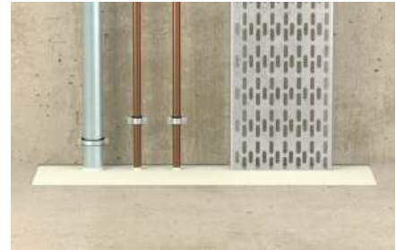
Mixed penetration through the floor
