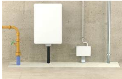
Mixed penetration through the floor
