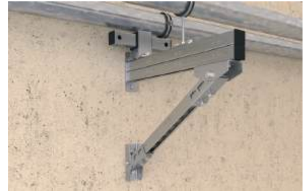
Massive bracing of cantilever arm
