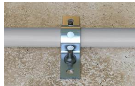
Fixing perforated tapes
