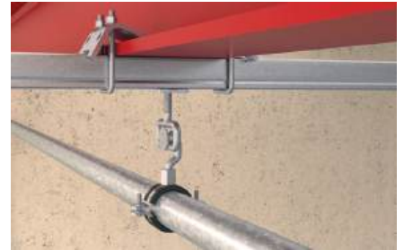
Channel to steelbeam
