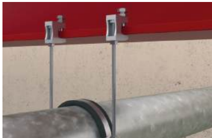
Heavy drainage pipe on beam clamp
