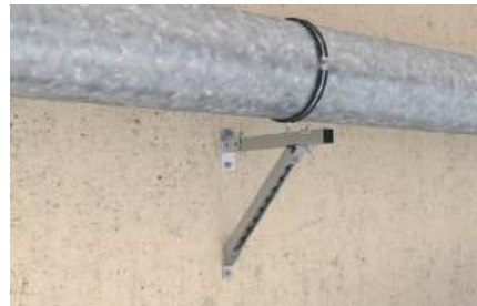
Spiral airduct on cantilever
