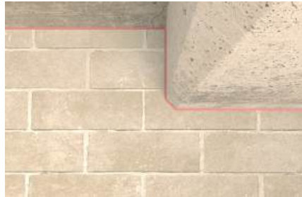
Construction joint application
