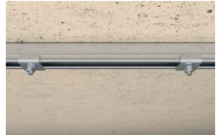
Channel installation at ceiling
