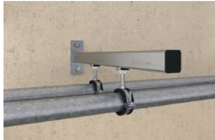
Light pipe fixing
