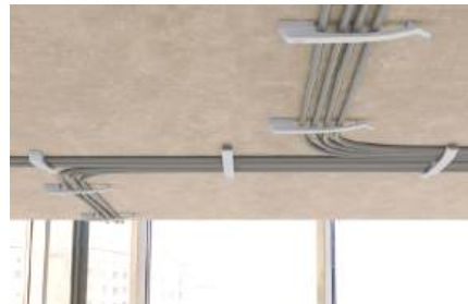
Fixing cable harnesses
