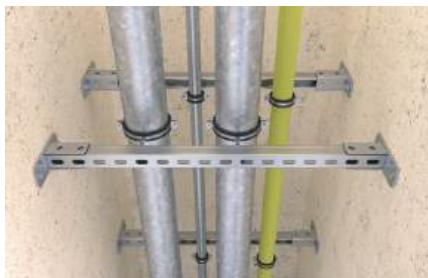
Pipe installation in escape route
