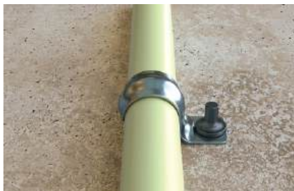
Fixing armoured conduits
