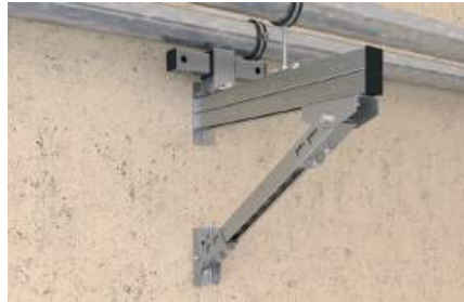
Massive bracing of cantilever arm
