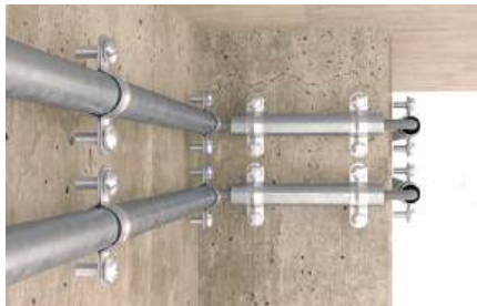
Fixing steel armoured conduits
