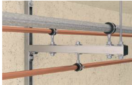
Cantilever construction with channel
