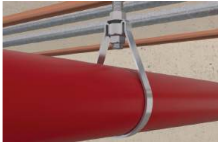
Sprinkler pipe installation
