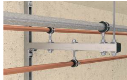
Cantilever construction with channel
