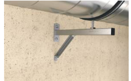
Ventilating pipe fixing at the wall
