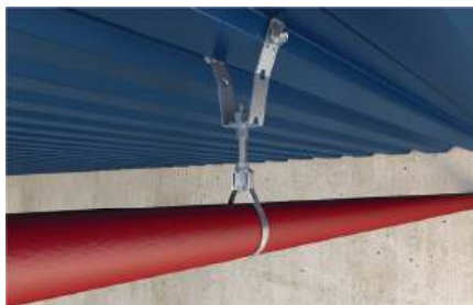
Sprinkler pipe installation to trapezoidal metal sheet
