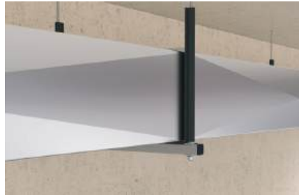
Air duct fixing with channel
