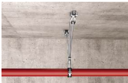
Bracing of pipeline with threaded rods
