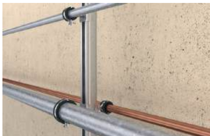
Lateral pipe mounting at channel
