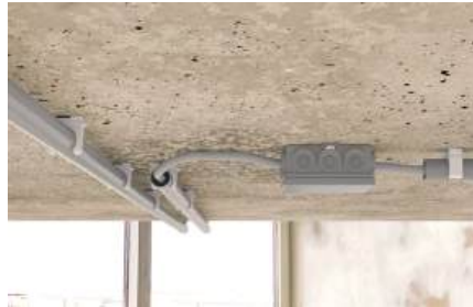
Fixing plastic insulating conduits
