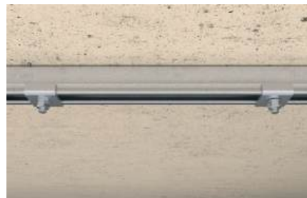
Channel installation at ceiling
