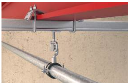
Channel to steelbeam
