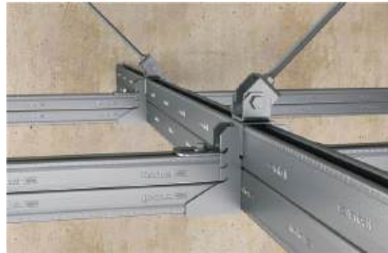
Inclined bracing for installation grid
